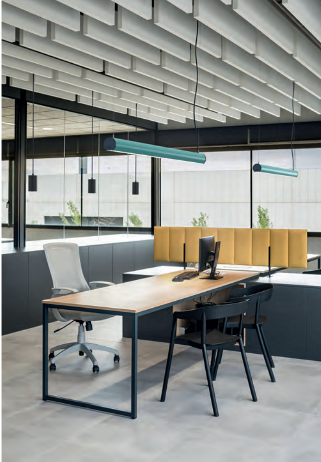
Spaces with hidden installations (acoustic louvred false ceiling).
